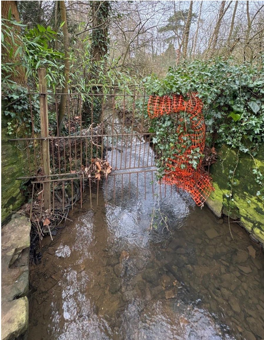
Figure 14 - Trash screen upstream of the footbridge (Source: Site visit Jan 2025)
