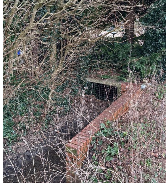
Figure 17 - Culvert inlet and trash screen in Ordinary Watercourse (Source: Site visit Jan 2025)
