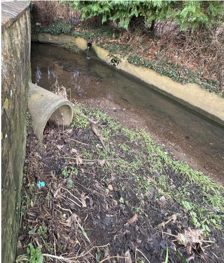
Figure 15 - Relief culvert outlet (Source: Site visit Jan 2025)
