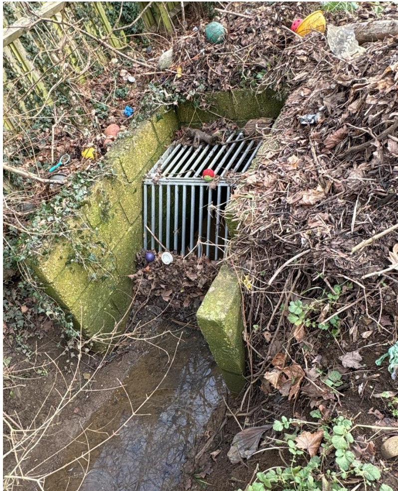
Figure 11 - Trash screen at culvert inlet near Bloxham Church of England Primary School (Source: Site visit Jan 2025)
