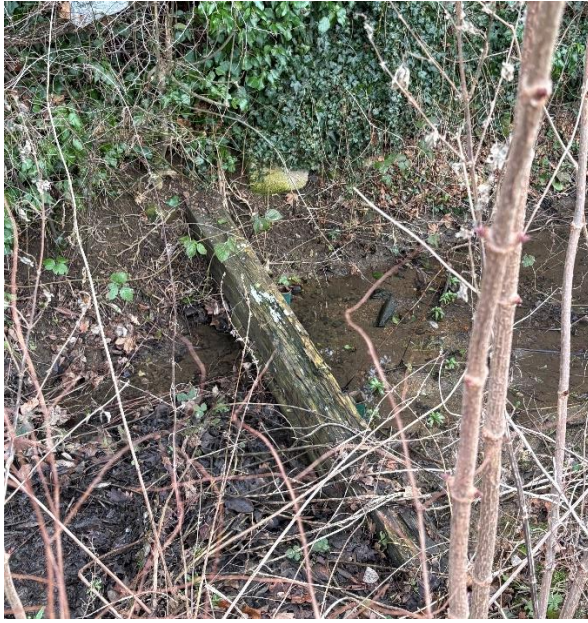
Figure 16 - Wooden baffle boards in Ordinary Watercourse (Source: Site visit Jan 2025)
