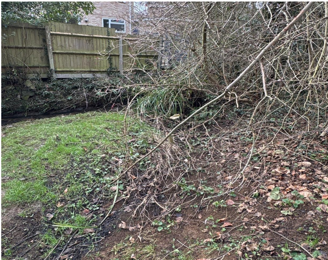
Figure 12 - Poorly maintained overflow route on Bloxham Brook left bank (Source: Site visit Jan 2025)
